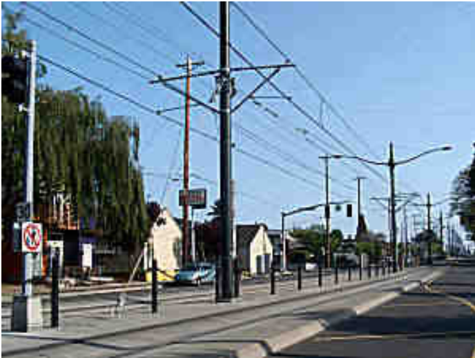
Ugly Overhead Wires
